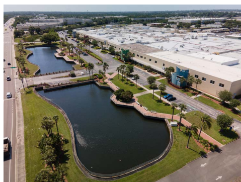
Aerial view of STAR Center
