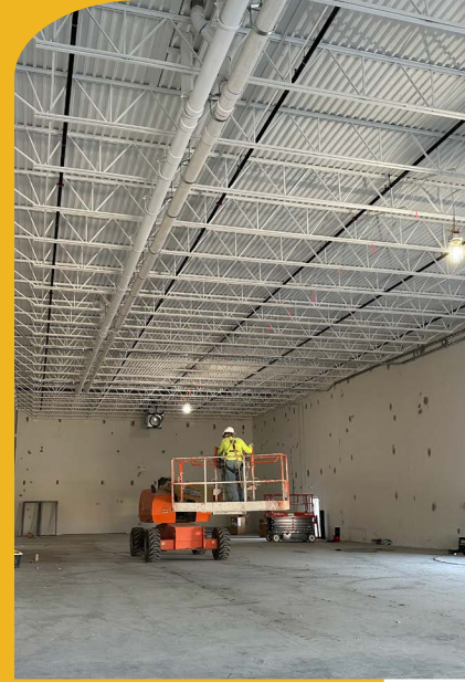
Pictured: AGORA Edge's new 47,900-square-foot facility under construction in St. Petersburg.
